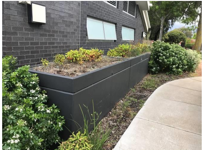
Raised bed / watertanks
