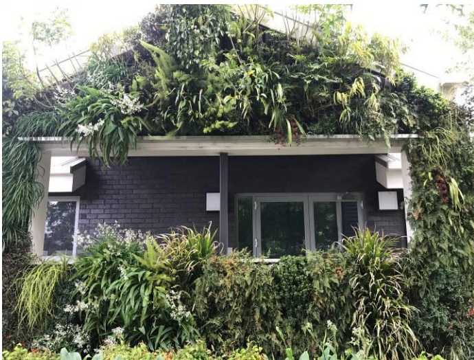
Front entrance vertical garden
